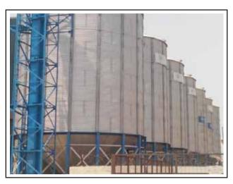
**SILOS FOR PADDY STORAGE** We have 7 silos for paddy storage each with capacity of 300 MT. Silos provide extra moisture free storage and helps to preserve paddy for a longer duration.
